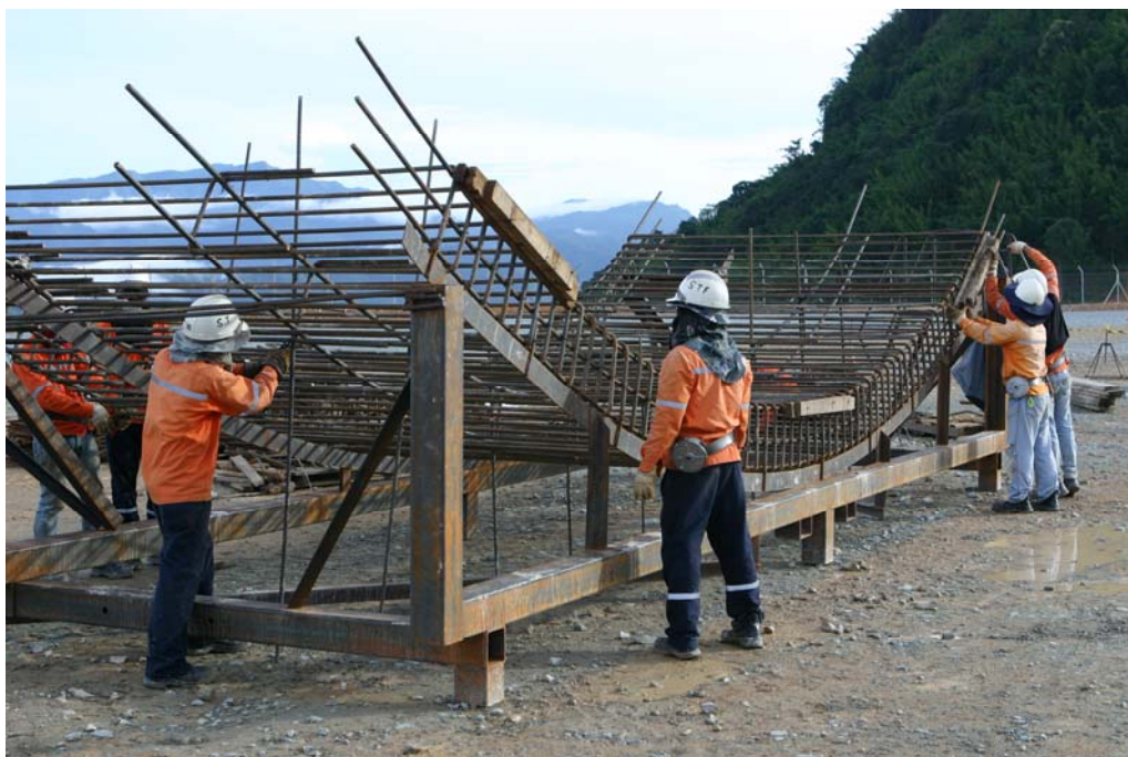
Construction of a pre-cast ringbeam for the CIL tanks
