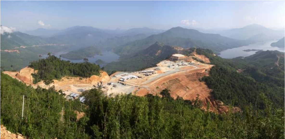
Ban Houayxai Gold-Silver Project site overview
