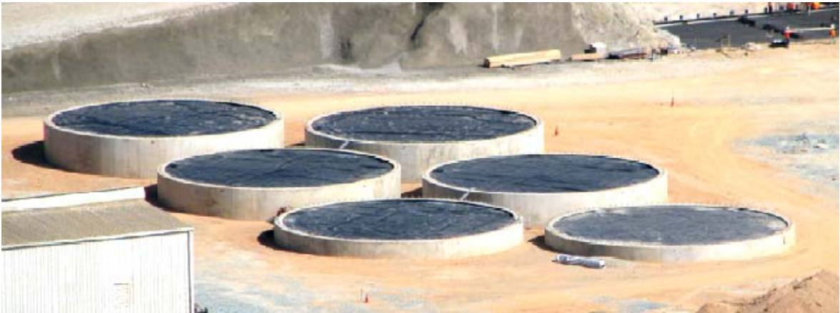
CIL tank ring beams installed and HDPE lining completed
