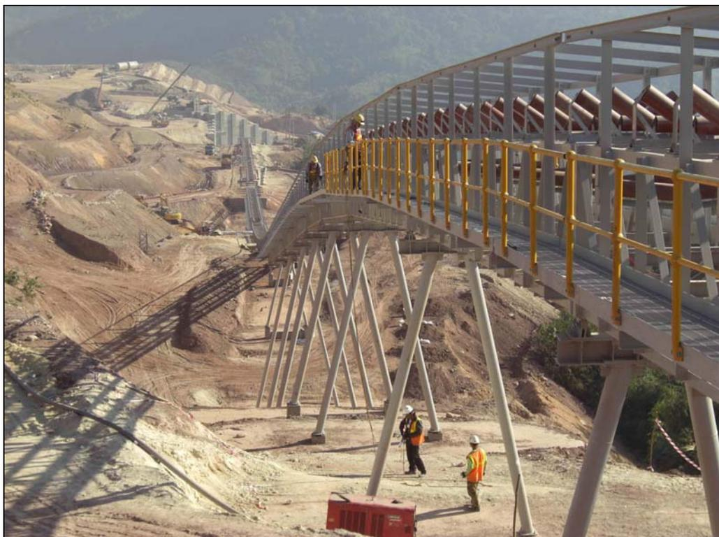
***Construction of the overland conveyor from the crusher***
