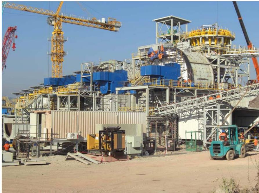
*Assembly of structural SAG and ball mill components completed and mills turned*
