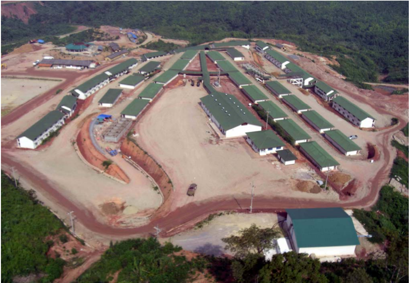
Phu Kham Operations accommodation
