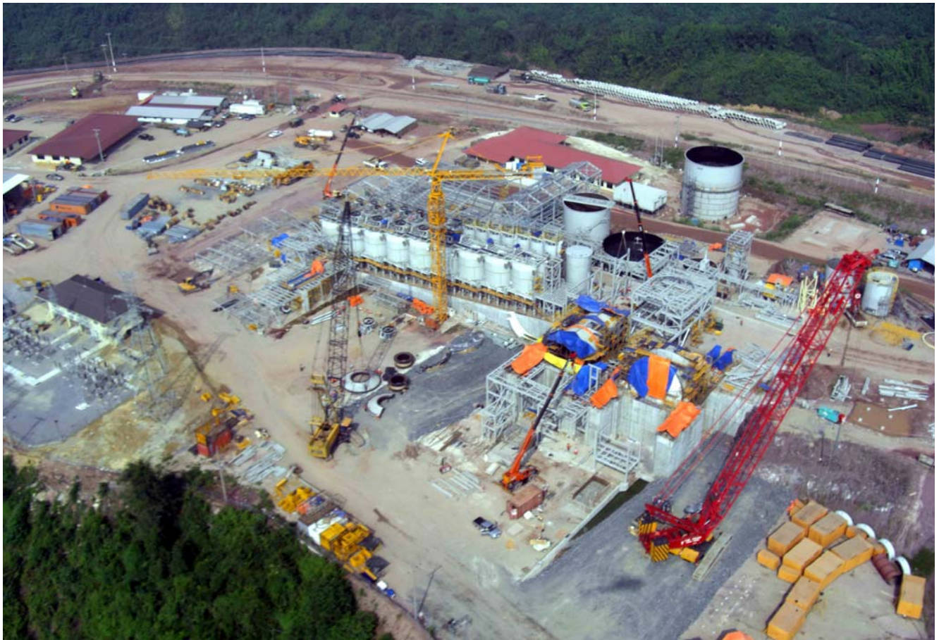
Aerial view of the flotation cells in position
