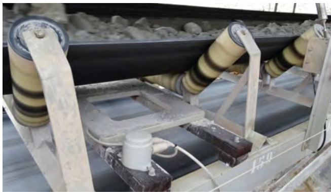
FIG 8 – SmartTag™ antenna installation under the semi-autogenous grinding feed belt.
