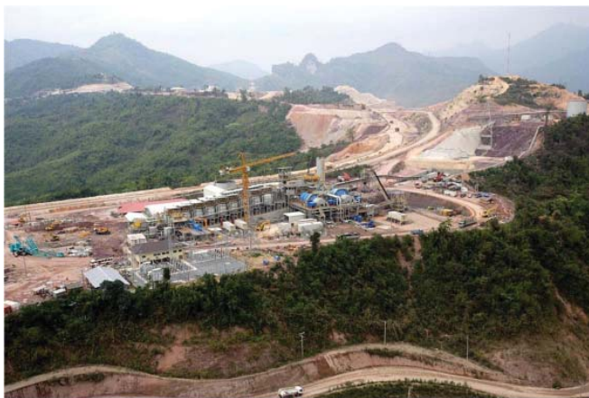
FIG 3 - Southern view of the Phu Kham concentrator, June 2008.
