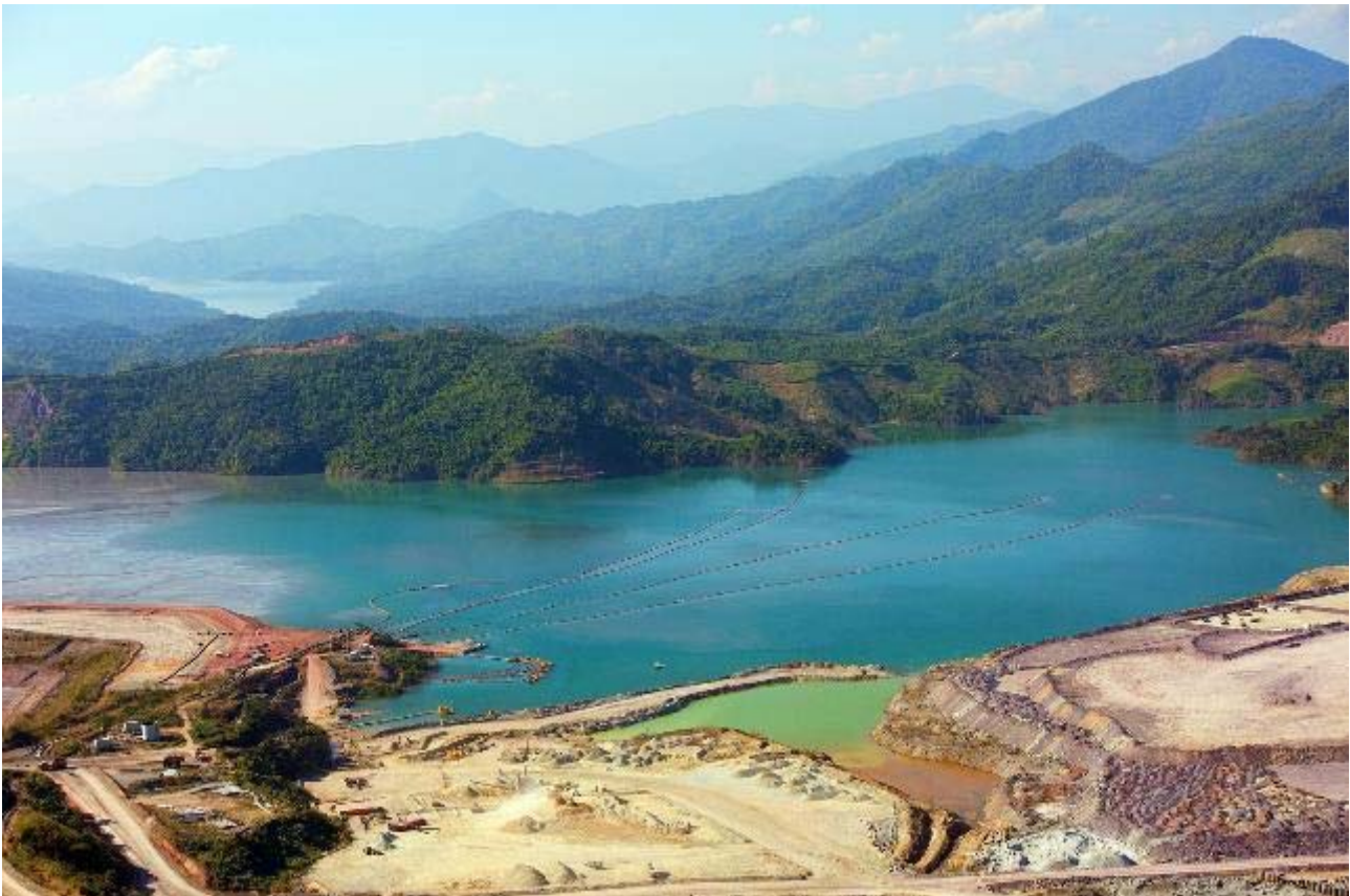
FIGURE 4 - Phu Kham TSF tailings pipeline deposition system with waste rock dump in lower right
