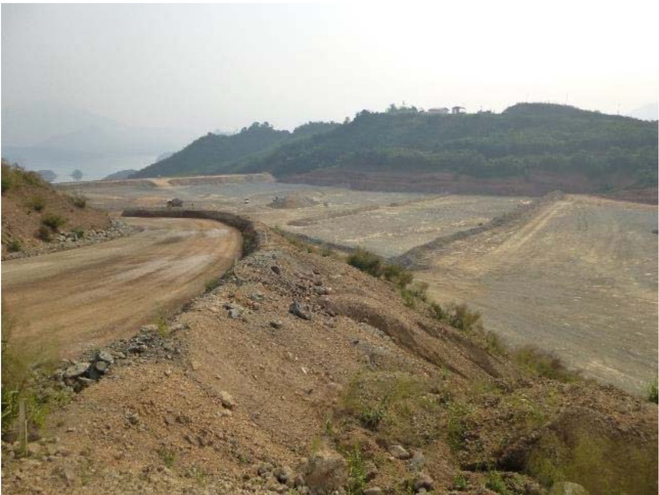
FIGURE 2 - Ban Houayxai waste rock dump construction
