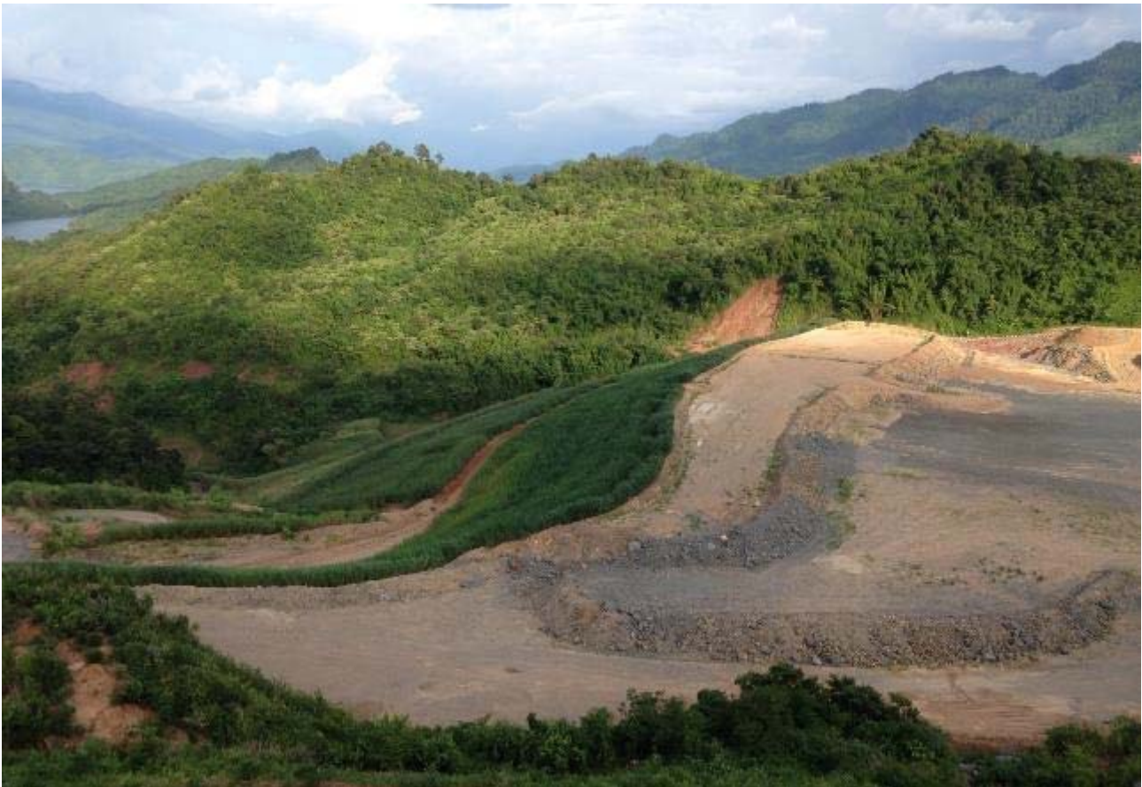
FIGURE 8 - Progressive rehabilitation of the Ban Houayxai waste rock dump
