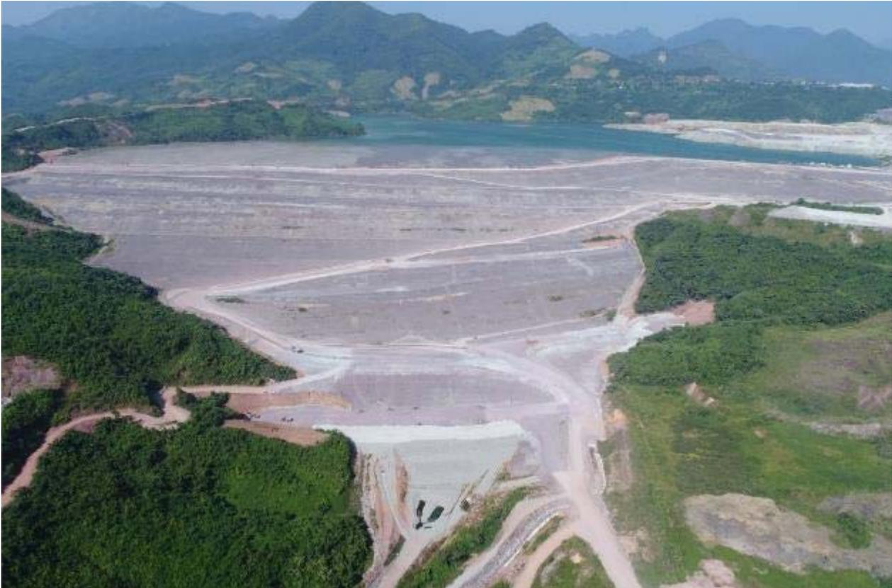
FIGURE 5 - Phu Kham TSF embankment downstream construction with waste rock dump in upper right
