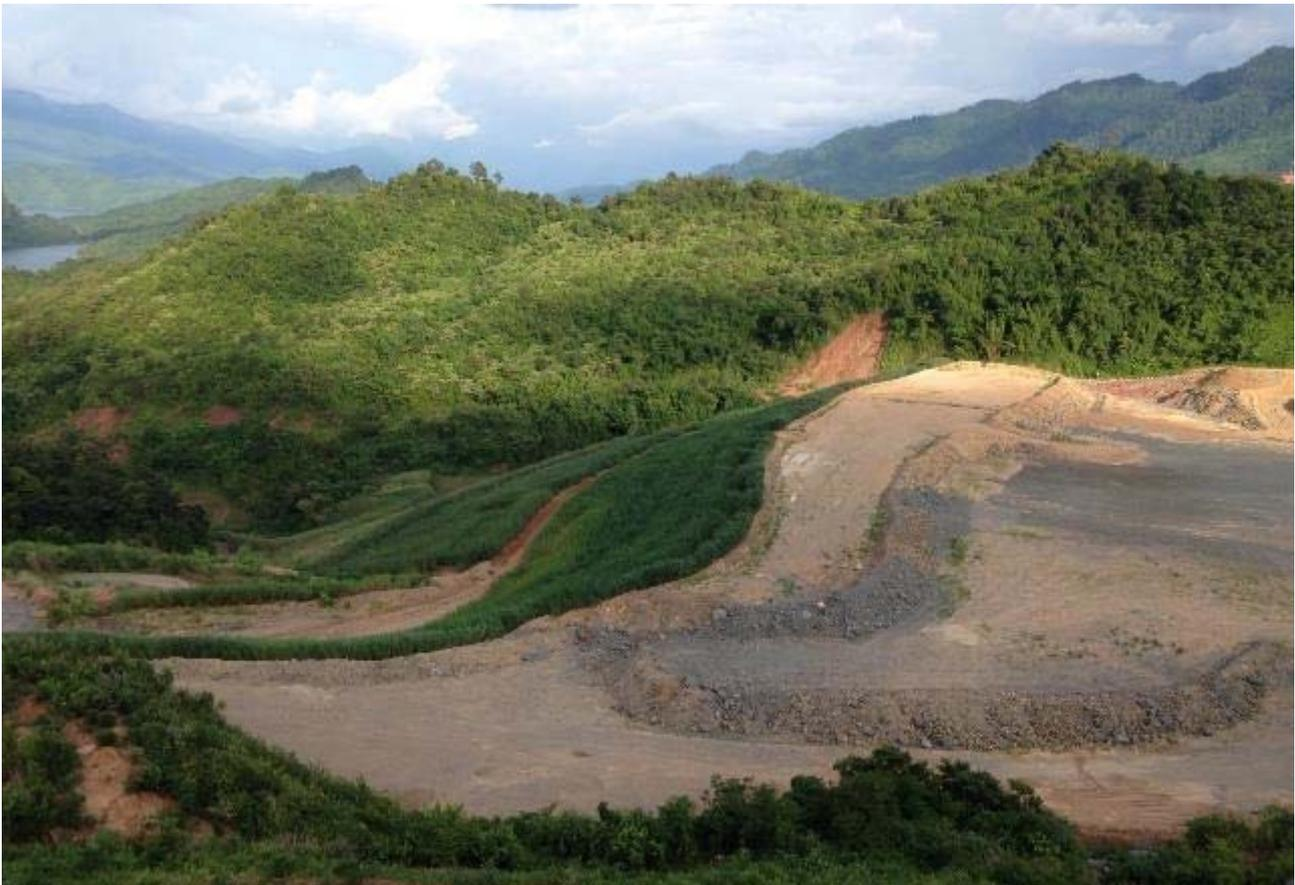
FIGURE 8 - Progressive rehabilitation of the Ban Houayxai waste rock dump
