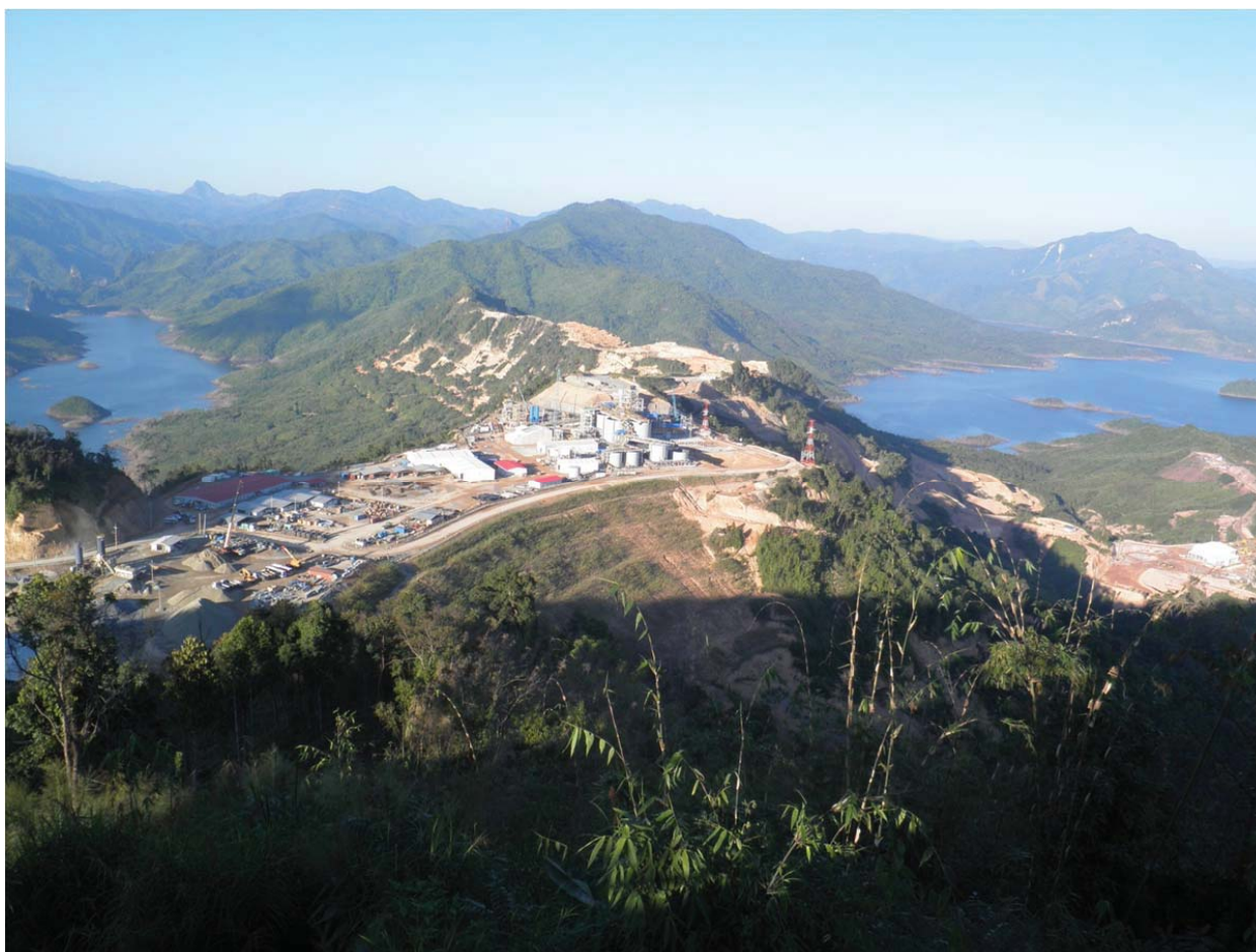
FIG 4 - Ban Houayxai project under construction January 2012.
