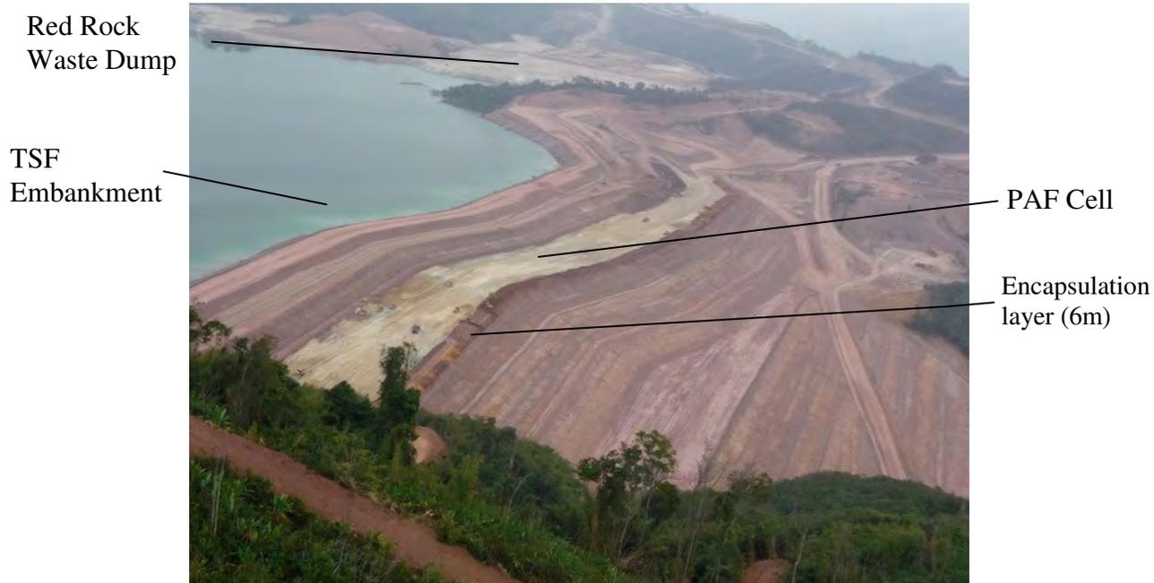
Figure 4: TSF embankment showing location of PAF cells in the downstream section of the dam wall
