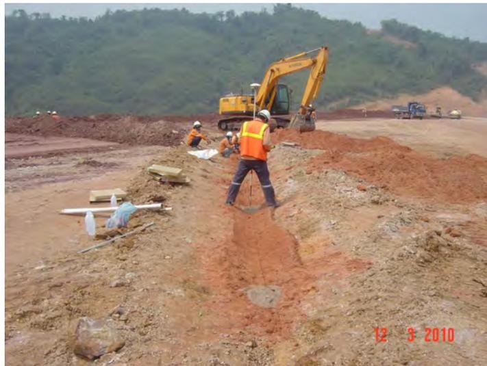
Figure 6: Installation of horizontal pore gas monitoring system
