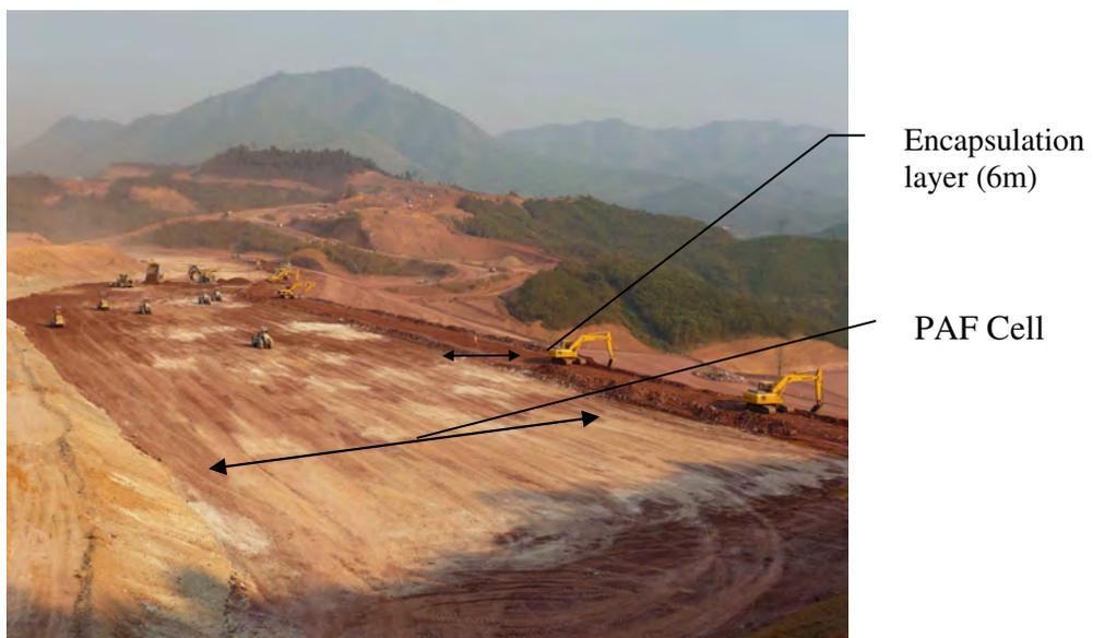
Figure 5: TSF embankment and PAF cell construction
